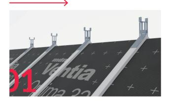
After previous placement of roof underlay and counter-battens, at the top of the roof there should be installed a BL (sheet metal) (or GW – nail) type ridge batten grip. The BL-type grip should be profiled accordingly.
